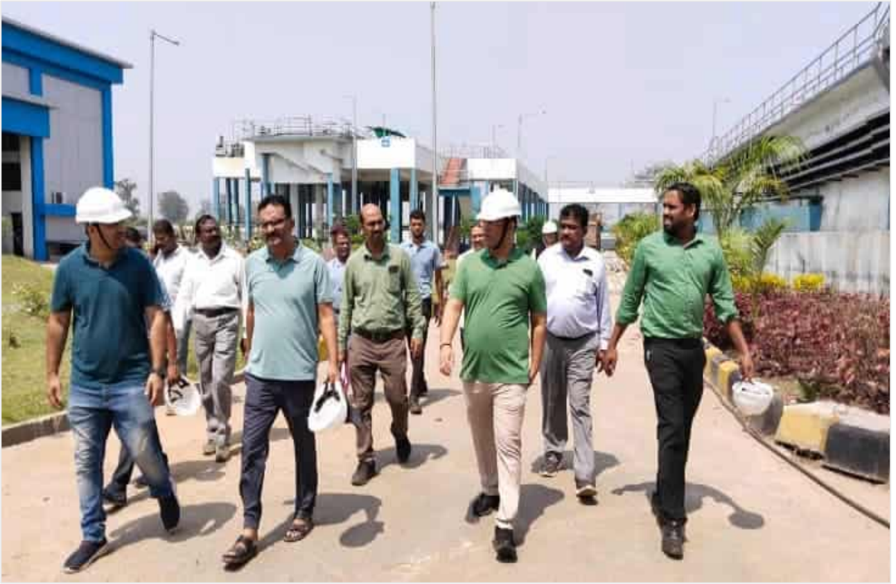
Chandandih STP in Raipur
