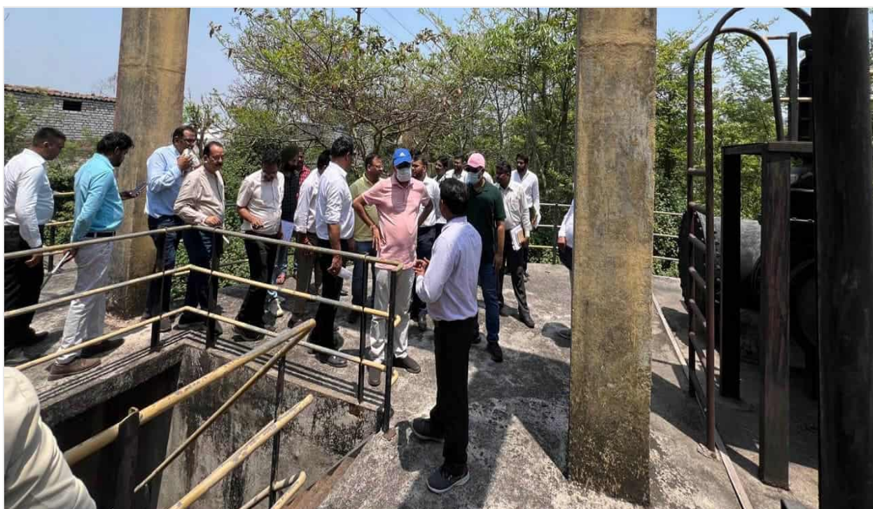
Domuhani STP in Bilaspur
