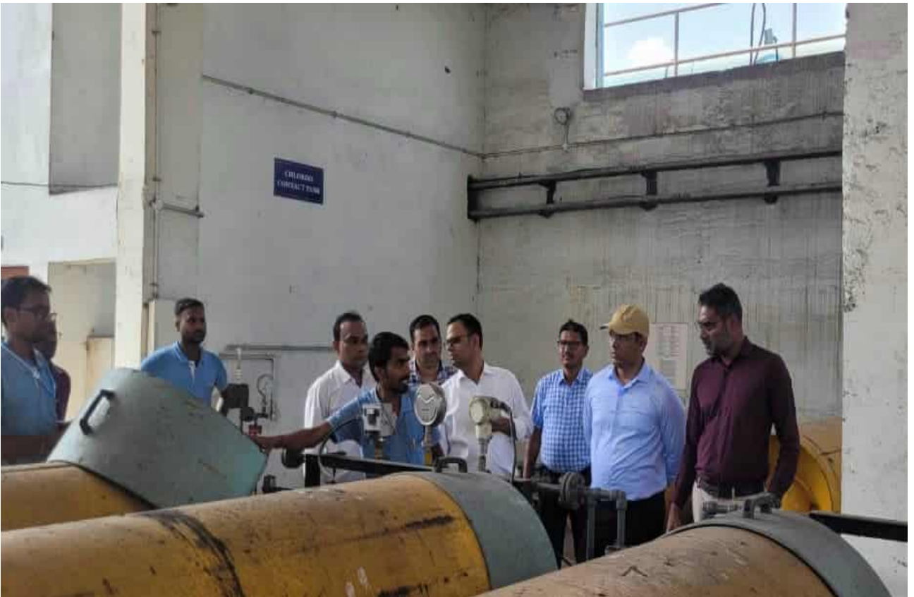
Nimora STP in Raipur
